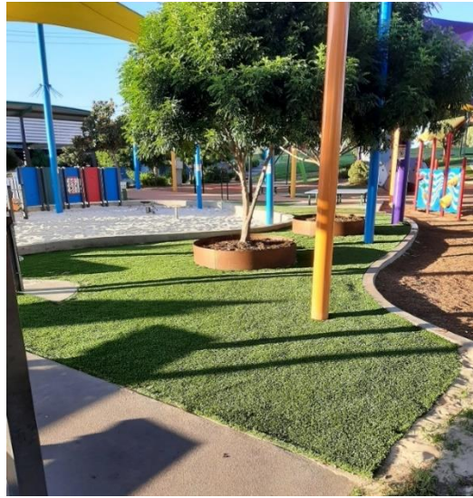
Regional Playground artificial turf installation in a high traffic area
